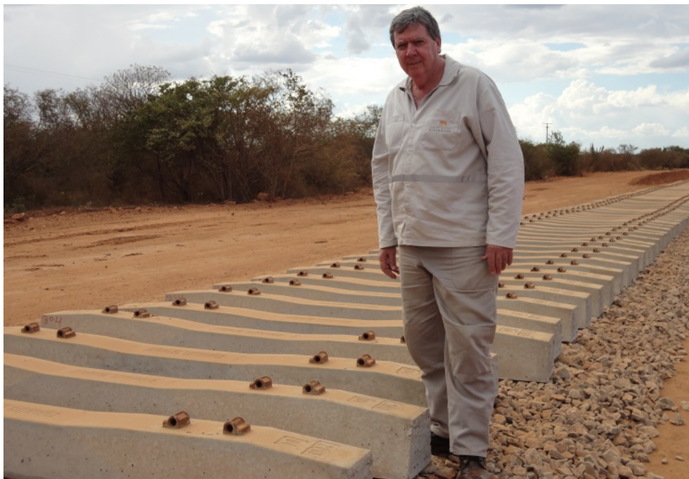
Figure 17-4: FIOL Railway Works Adjacent to the South of the Project Area
