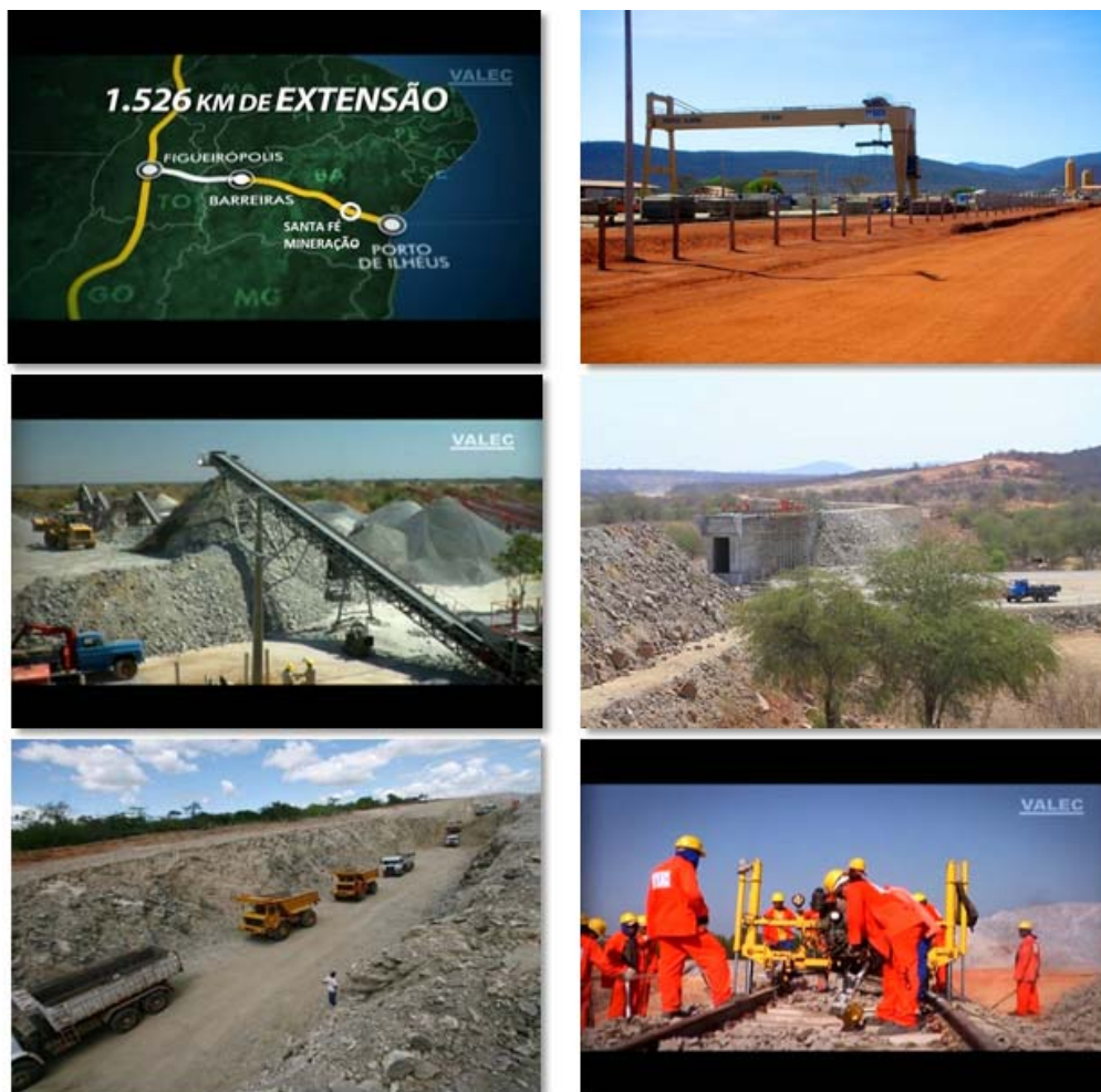
Figure 17-5: FIOL Railway Works
